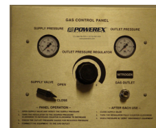
Gas Control Panel
