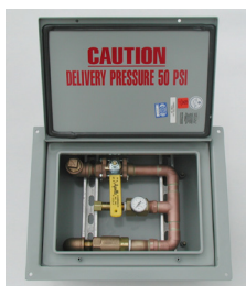
Emergency Oxygen Inlet Box
