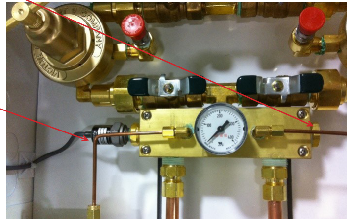
Emergency reserve low pressure transducer (14-3001-12) installed into port on RWP reserve manifold by plumber.
