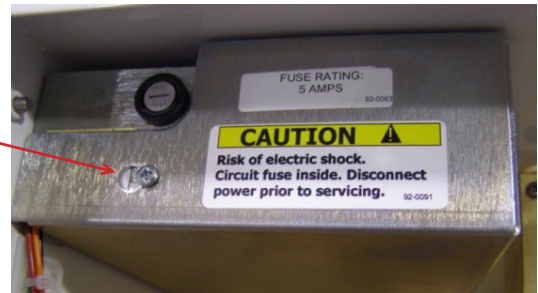
Conduit knockouts for 120 VAC Conduit knockout for low voltage alarm signals
