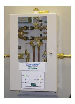
The control panel shall incorporate a set of LED's for each bank, green for "Bank in Use", amber for "Ready" and red for "Empty". Analog gauges are also provided so that line and both bank pressures may be observed.
