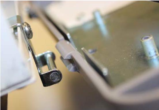
Attach the two (left & right side) lanyard cables to the alarm back box and (if necessary) front panel using the screws provided.
