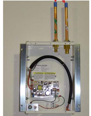
After removing the protective plastic caps, connect the riser extension tubes to the gas piping system per NFPA 99. Make sure the drop is for the proper gas service. Using a purge gas to insure cleanliness in the tubes, silver braze the joints. **Do not use soft solder.** Conduct heat away from the check valves. (Per NFPA 99 Chapt 5 a nitrogen purge is required). The 150 psi standing pressure test of the piping system must be successfully completed and all pressure removed
