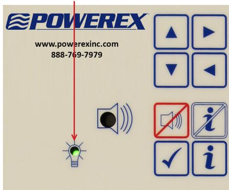
If you haven't already, you are now ready to pressurize the piping system to normal operating pressures. The alarm is shown here with Medical Vacuum at normal operating pressures. All remote signal points (master alarm signals) are shown in normal condition.
