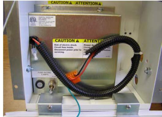
To remove the power supply cover, loosen the two screws at the top of the cover and slide the cover to the right, then lift the cover over the screw heads. Slide the wiring harness strain relief to the left until it is free from the cover.
