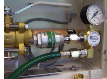
Dual port EZ Backfeed™ fitting with Gauge, transducer, and back-feed hose attached to DISS gas specific demand valve shown above.
