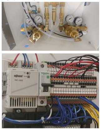
Connect the final line hi/lo pressure switch wires to the correct location. There is a 12" length pair of low voltage wires with a near the PLC with a lever nut on the end. Make sure the wire is routed in a way that the manifold cabinet door can open without stretching the wire.
