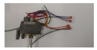
Connect the Emergency Reserve transducer and pressure switch to the correct terminal block near the PLC. The transducer and pressure switch are both installed on the emergency reserve regulator.
