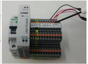
It is important that the sensors are wired to the correct terminal block. Per NFPA 99, an alarm will sound for cross-connected sensors.
