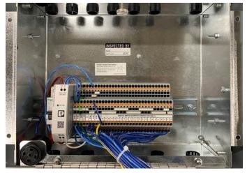
Rough-in box contains power supply, circuit breaker, terminal blocks, input expansions and holes for main line power connection and riser connections.
