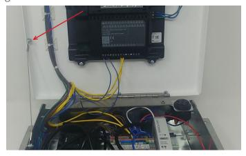
Plug wired connectors from terminal blocks into appropriate input blocks in PLC.
