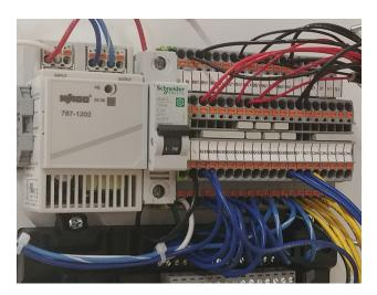
Connect the final line hi/lo pressure switch wires to the correct location. There is a 12" length pair of low voltage wires with a near the PLC with a lever nut on the end. Make sure the wire is routed in a way that the manifold cabinet door can open without stretching the wire.
