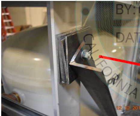
Brace attachment detail
