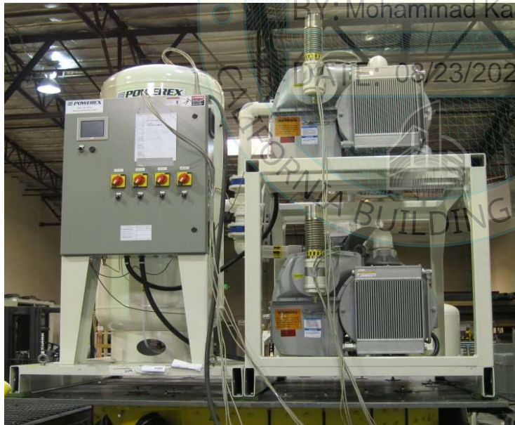
UUT2, view from front
