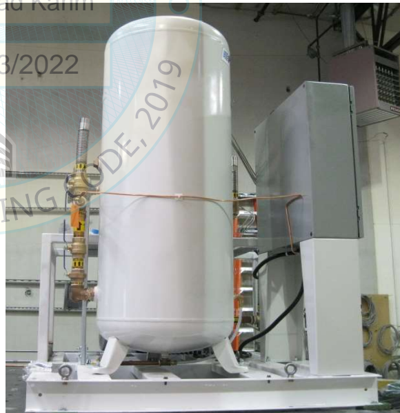
UUT1, view from left
