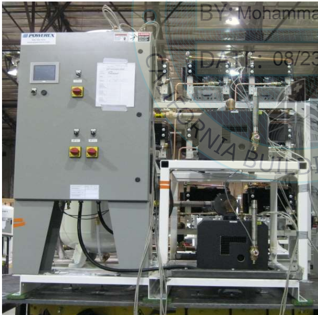
UUT3, view from front
