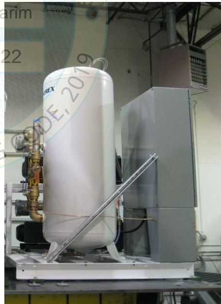
UUT3, view from left
