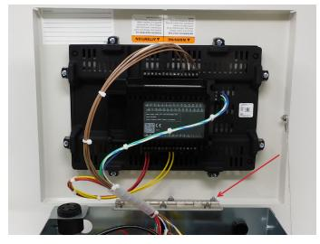
Place unattached side of panel lanyards over provided threaded studs on the left side of the cover assembly. Place provided washer and hex nut over the stud and tighten the hex nuts.
